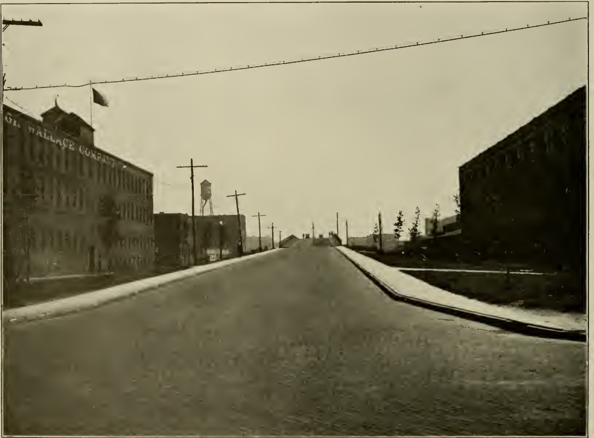
Viaduct, East Grand Boulevard, Detroit, Michigan.
